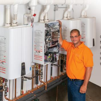
Contractors recommend Navien for its stainless steel heat exchanger. "It will last a lot longer than copper heat exchangers on other tankless units."
